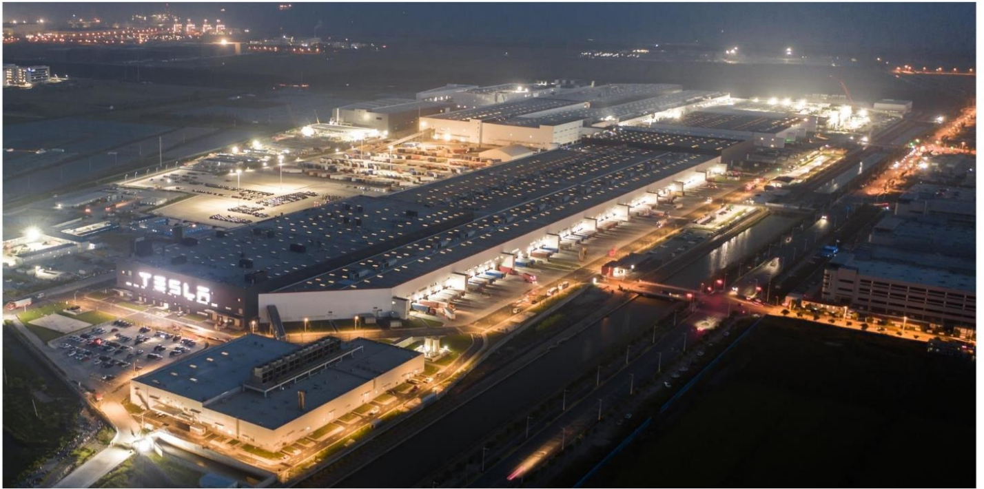
GIGAFACTORY SHANGHAI - MODEL 3 FACTORY (FOREGROUND); MODEL Y FACTORY (BACKGROUND)
